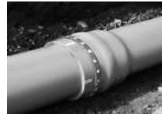
Pin-and-Groove Gasketed Joint
