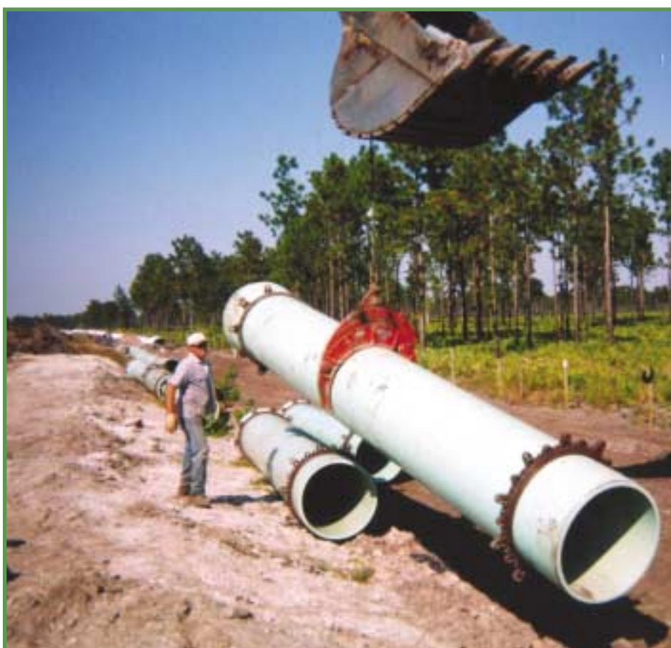
30-inch PVC was installed for the wastewater force main.
