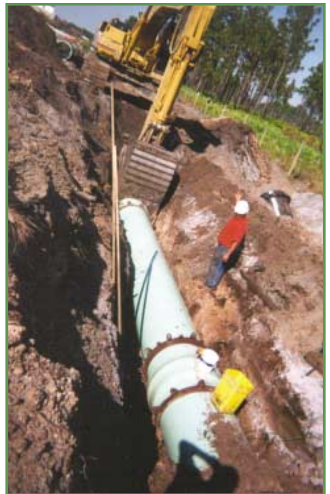
An average of 500 feet of pipe was installed per day.
